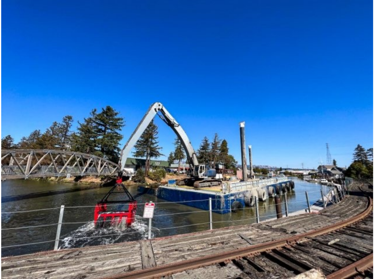
Figure 1: Clamshell Dredging Near the Trestle and Balshaw Bridge in the Turning Basin
