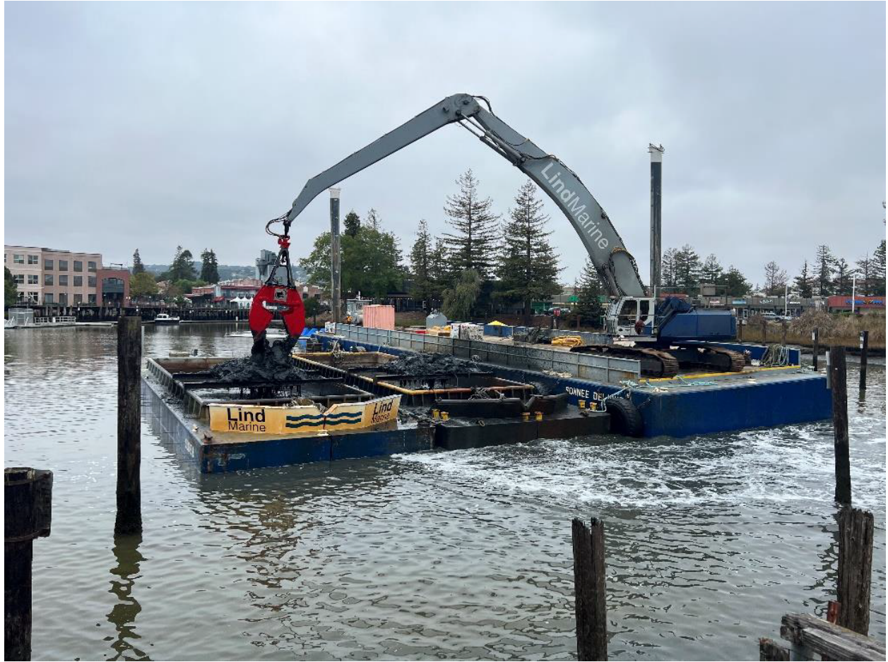
Figure 2: Turning Basin Dredging – Loading Scow for Transport to Designated Deposit Site
